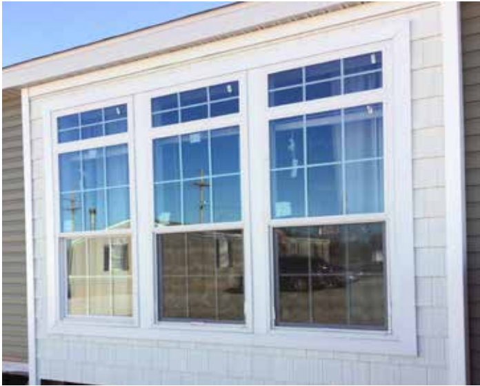
B-297 with Transoms and Shake Siding
